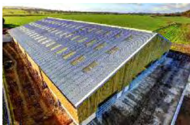
Ashdowne Grange Farm, using Profile 6 with spaced roof ventilation system
