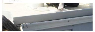
Make sure the laminating roller is used in a controlled fashion (slower) so as not to generate spray.
