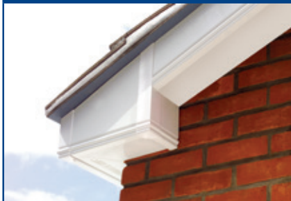
Box End Detail 2: Mammoth Board fascia, bargeboard, and box end cut from a section of fascia.
