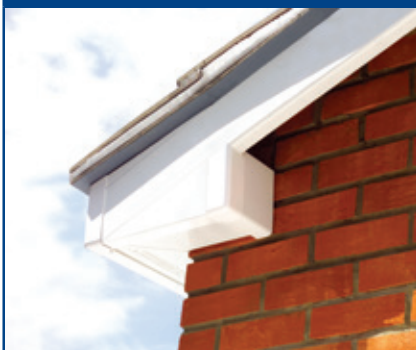
Box End Detail 5: Bargeboard extending to meet the fascia.
