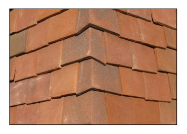
12 The finished external corner should be a best fit with the external angle tiles sitting together with minimal gapping, and unable to rattle.
