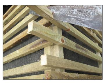
At the first external corner the 38 mm x 25 mm battens running up to the corner should be left long, and the adjacent batten running away from the corner should be butted up to the batten that has been left long, levelled and fixed into position. The excess batten should be cut off flush with the face of the batten on the adjacent wall face to produce a neat square corner ( no gaps).
