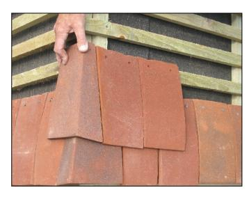
Proceed to install the first full course of plain tiles working to the chalk lines marked on the battens. The chalk lines should either be the side of a tile or the centre of a tile. Tiles will need to be adjusted to even out the gaps and wide tiles may need to be rejected, moved, or trimmed to make them fit. Lay the full row before attempting to install the first external angle tile. Do not nail the end two tiles as they will need to be cut to fit.
