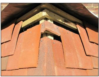
11 If in the course of the work an external angle tile is broken, and needs to be replaced. The tiles above in a large V must be stripped down to the broken tile, the broken external angle replaced and the tiles reinstalled and fully nailed back up to the top edge or gable. The use of mastic, or homemade wire or metal contraptions to hold the replacement external angle tile in position, will not be acceptable.
