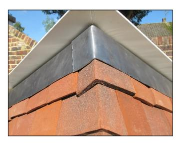
10 At a top edge the final external angle tile will need to be cut drilled and fixed to the top tile batten to match the top tile course, either up under a soffit board with a lead cover flashing, or above the soffit board line to hide the top line of tile fixings. Where there is a gable end meeting a soffit on an external corner, the top tiles will need to be mitred rather than a cut down external angle, as the cut on the gable side of the corner will be a Winchester cut.
