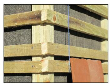
5 Starting at the right hand eaves, lay out the first row of full tiles and repeat at the top edge abutment with the soffit, and using a chalk line ping vertical lines up the battens to coincide with the side of every 5<sup>th</sup> tile. To achieve a vertical line the eaves or top course may need to be adjusted.
