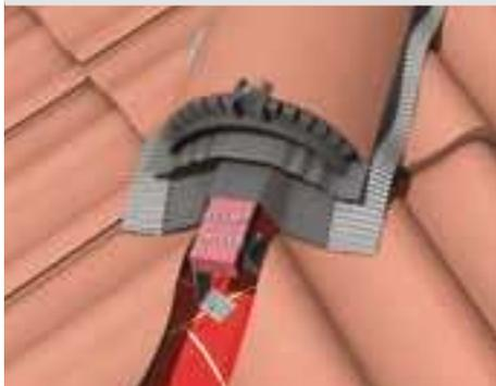
Simple and rapidly installed ventilated dry hip system, compatible with all tiles and slates up to 45° (suitable up to 60° subject to tile/slate profile and hip tile type).
