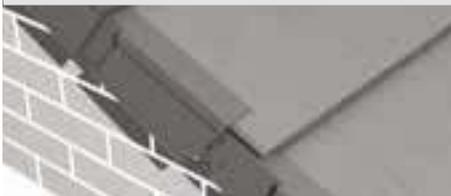
Compatible with Edgemere, installed at a range of headlaps and rafter pitches from 17.5-45° (suitable up to 55° when used with the 'steep pitch ridge batten section', see Dry ridge system).
